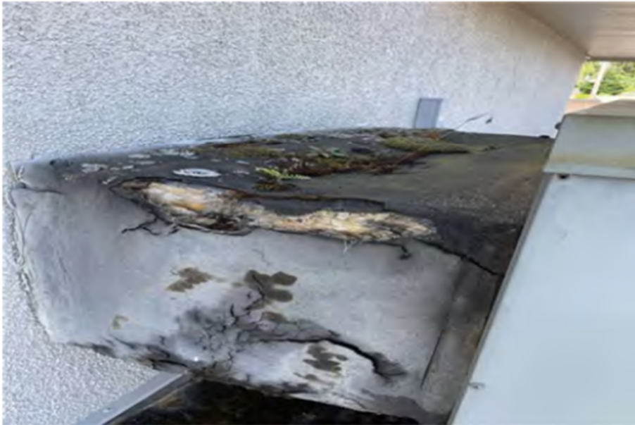
Insulated vent from HVAC to wall in poor condition.
